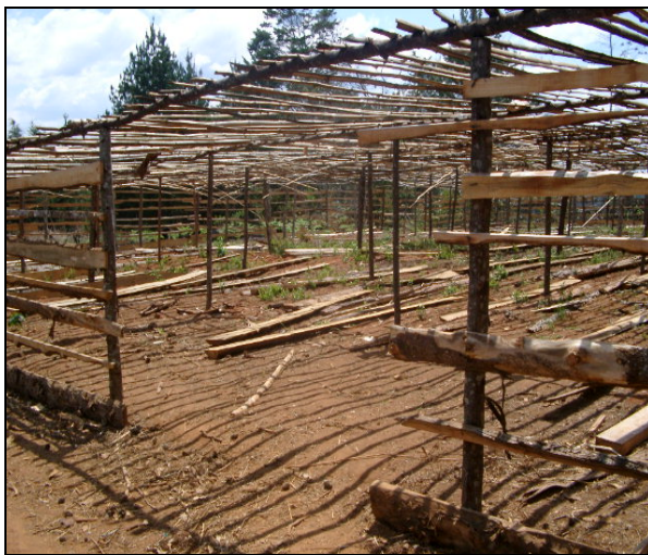
Plate 2: Initial stages of a nursery shed construction
